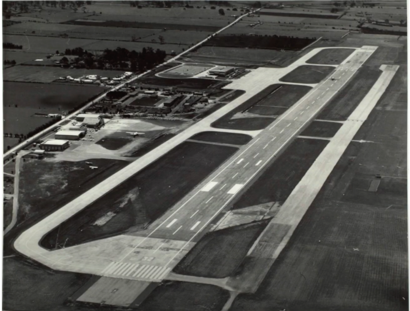
Tasmanian Aviation Historical Society (1967) Runway commercial expansion and Terminal under construction
